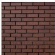
6. RESTORED FACE BRICKWORK
